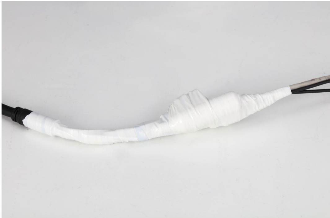
Figure 1-3 Covering exposed parts
